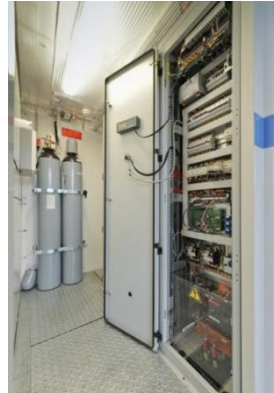
Container with ancillary systems
