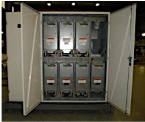
Interchangeable Rack Mount Power Converter Modules Allow for Easy System Configuration
