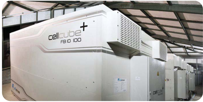
3x FB 10-100 CellCubes at Indian Customer site
