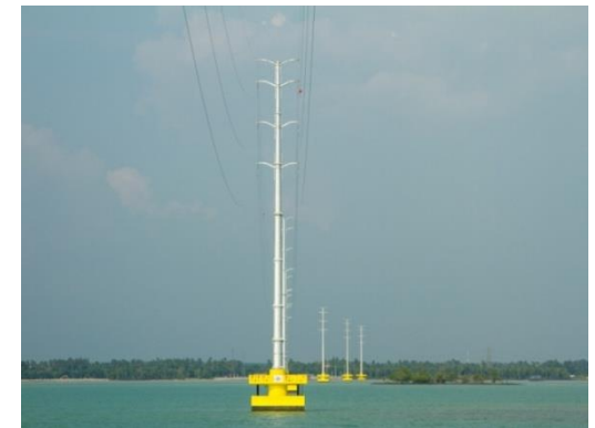
Typical Poles located in a River Crossing
