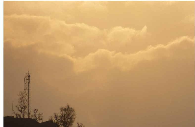
BTS tower – 0.8 kW
