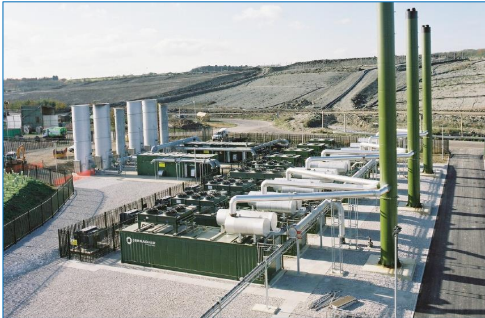
Biogas engines and flares installed at Brogborough landfill site, UK and Bisasar Road landfill site, South Africa
