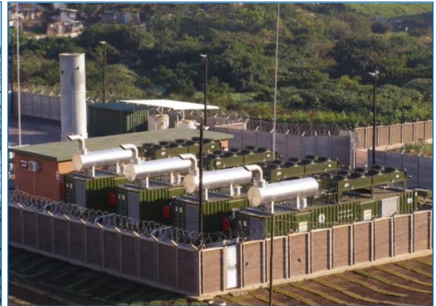
Biogas engines and flares installed at Brogborough landfill site, UK and Bisasar Road landfill site, South Africa
