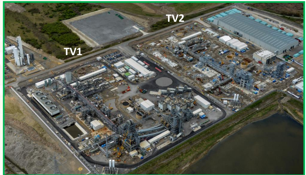
WPC Gasifier and Auxiliary Modules installed at TV1
