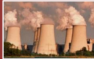
Coal power plant
