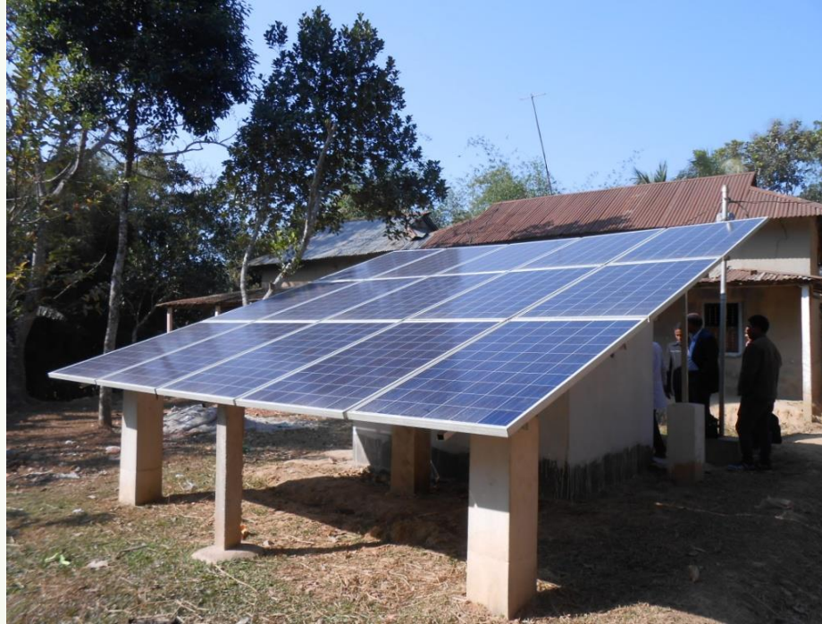
Fig. 4: A Pilot three kW p Solar PV system installed at Baroihati near Kapashia, Bangladesh.
