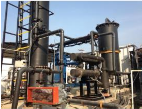
Raw Biogas Refinery
