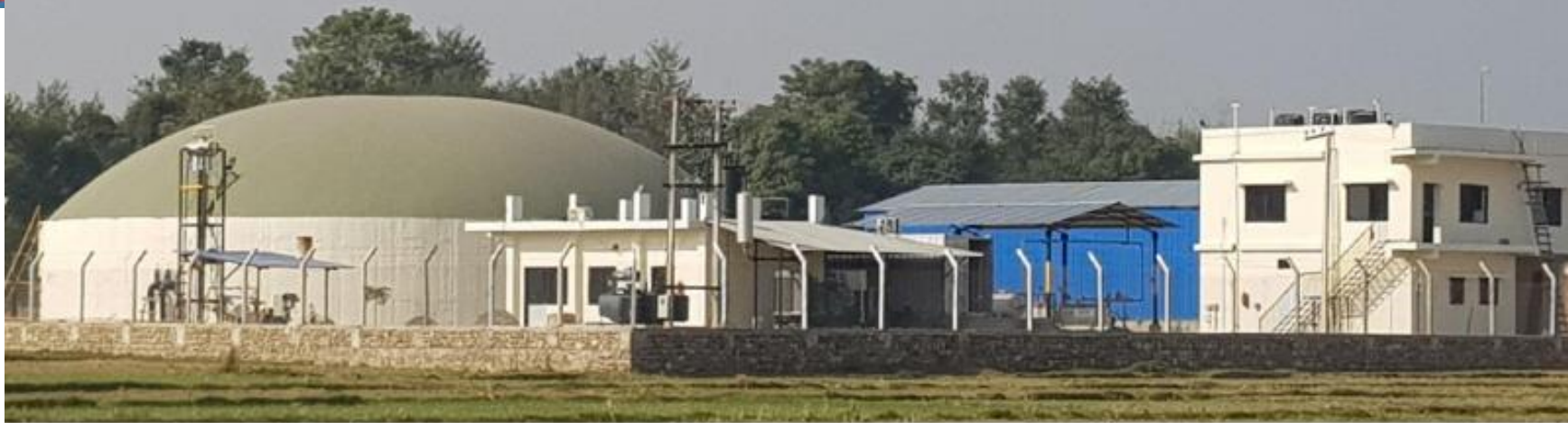
Biogas plant and other facilities
