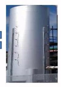
Single 6m x 2.4m storage unit normal charge stores 29.92MWh thermal
