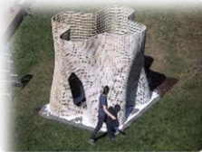
UC Berkeley unveils first-of-its-kind 3-D-printed cement structure
