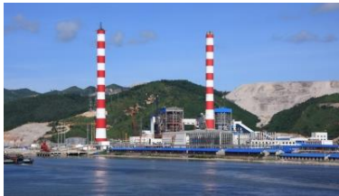
Coal Power Plant
