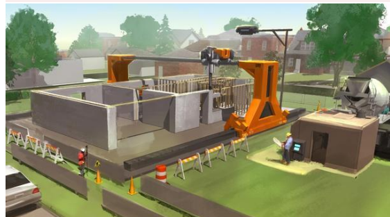
Utilizing high-performance fast-curing cement material for 3D printing construction
