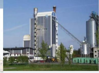
Electricity: 6 MW District heating: 9 MW (overall efficiency: 94%)
