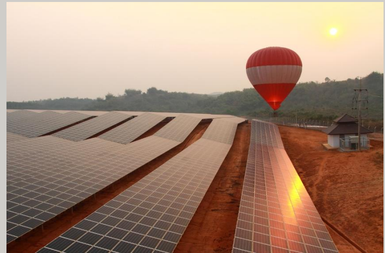
Solar PV farm in Thailand. Photo credit: Energy Storage News
