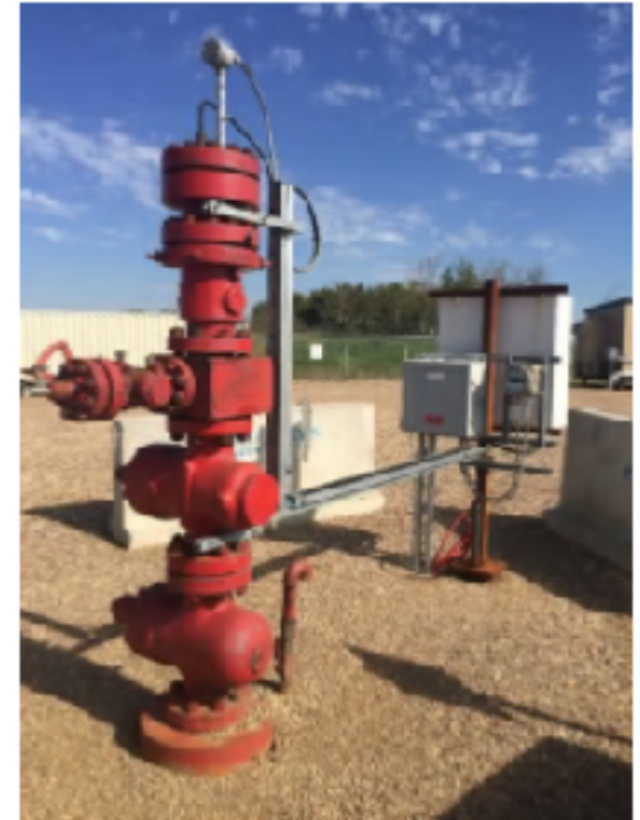
Monitoring well at the Quest CO 2 Storage site.
