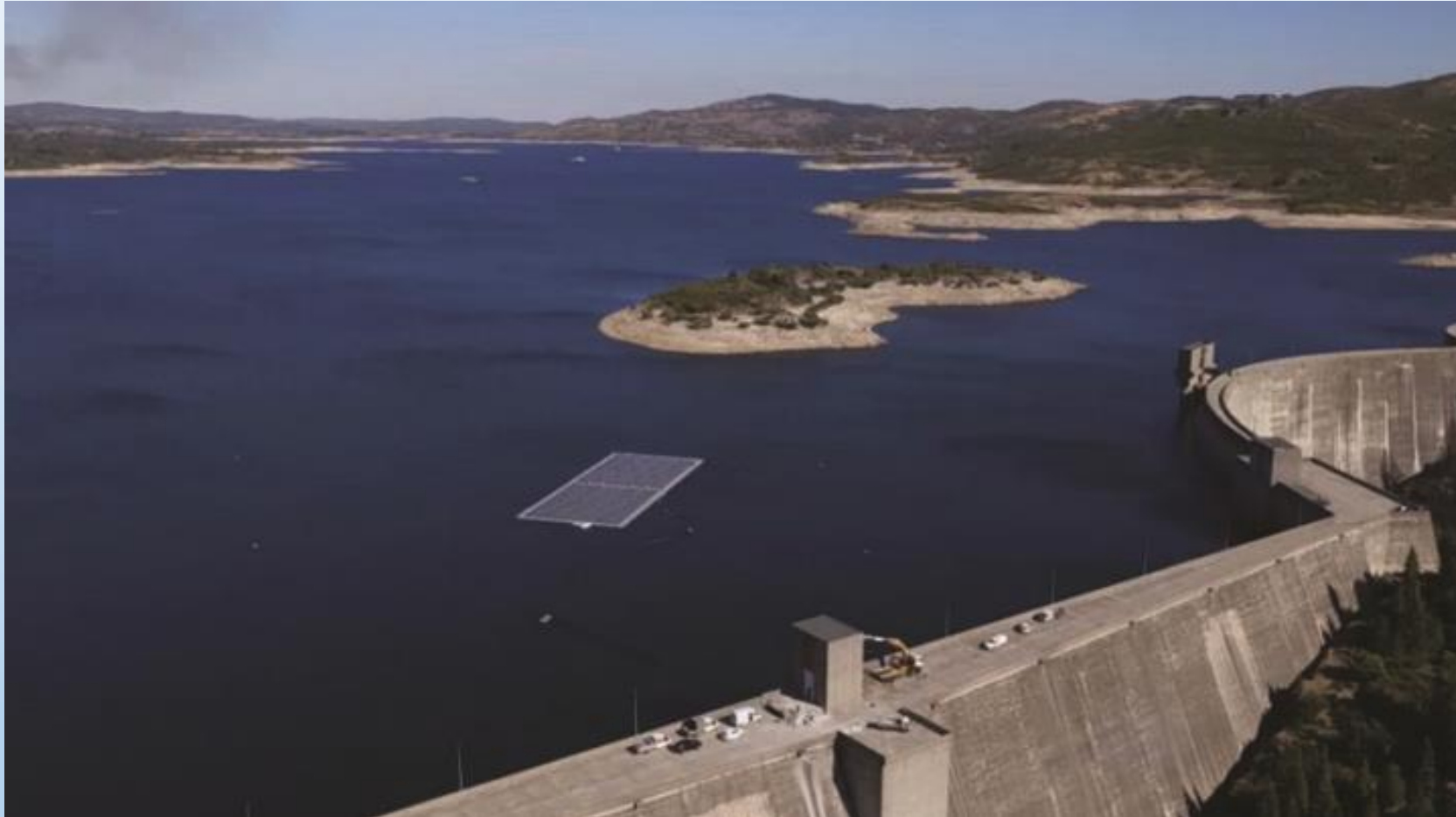
Alto Rabagão dam in Portugal: World's first floating photovoltaic project in which the solar power is integrated with generation from a hydropower plant. Floating Solar PV adds 220 kW to the 68-MW hydro plant
