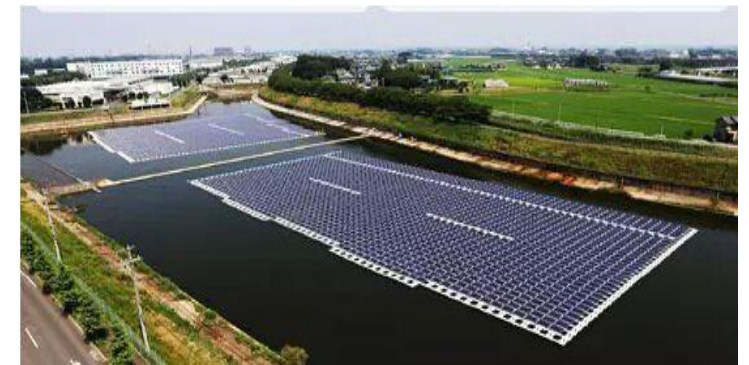
Trina Solar Okegawa Japan 1.2MW Floating Project
