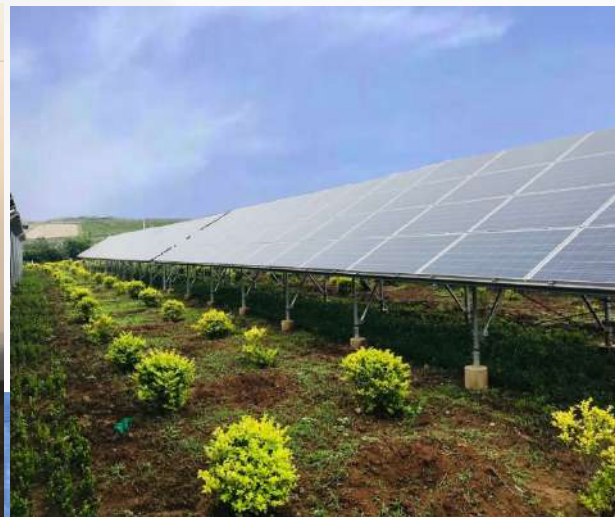
Shandong Wudi poverty-alleviation related PV Power Generation Subproject
