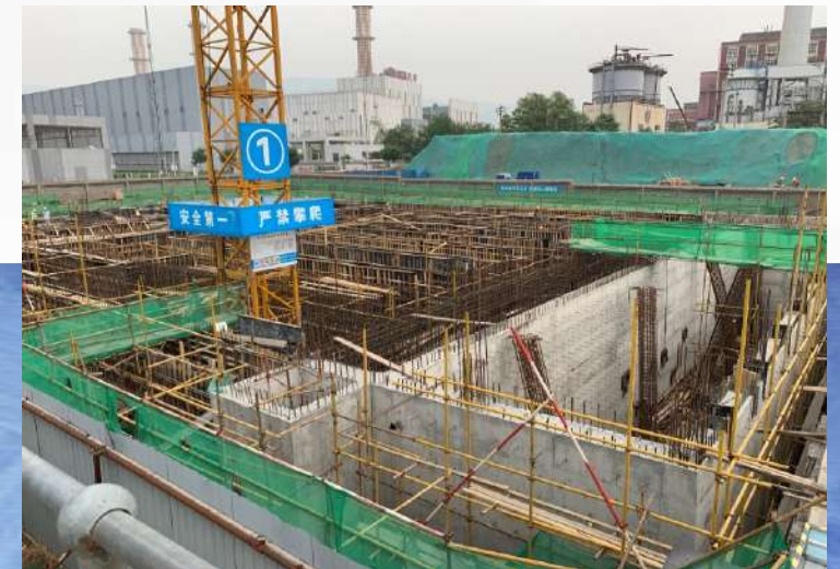
Subproject Construction Site
