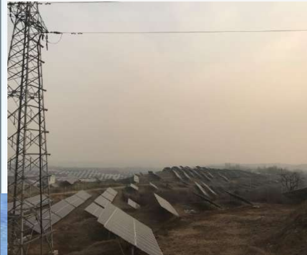
Hebei Xingtai Centralized Solar PV Power Generation Subproject
