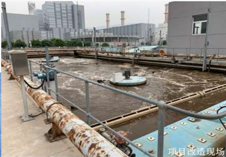
Subproject Reconstruction Site
