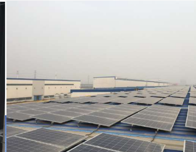
Henan NeihuangZhongguang Distributed Solar PV Power Generation Subproject
