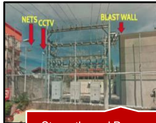
Strengthened Power System Resilience
