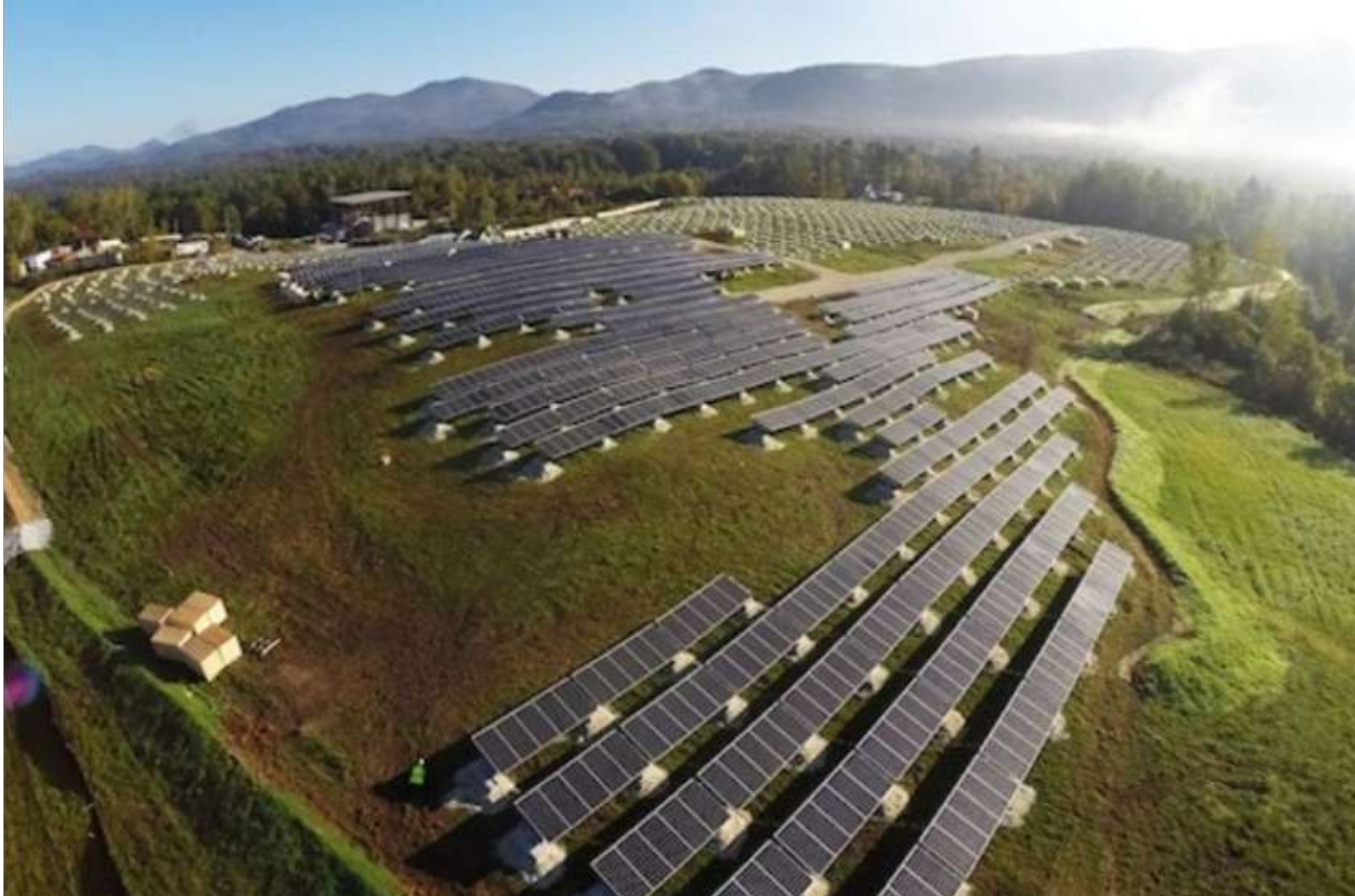
Source: Green Mountain Power, Stafford Hill
