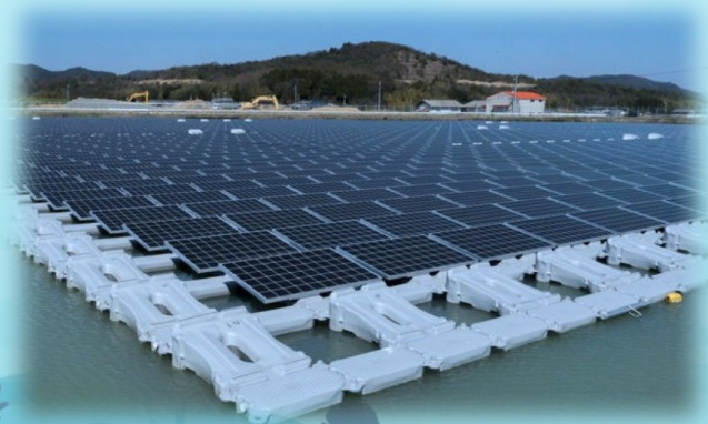
HDPE type (Source: Ciel & Terre)
