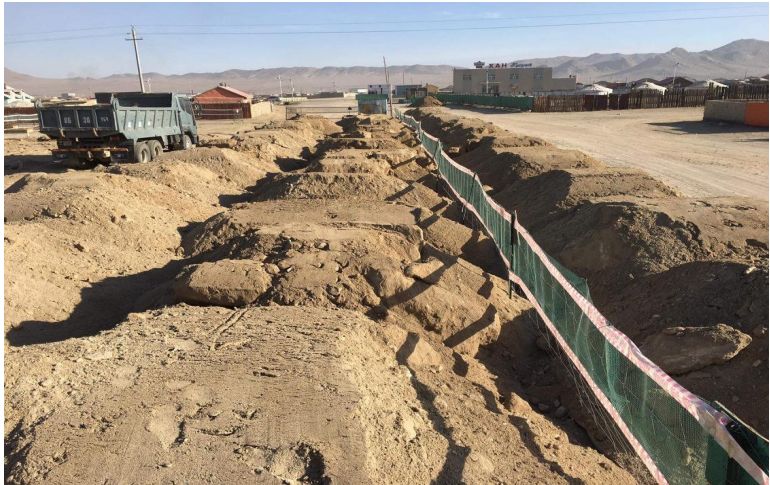
Kindergarten in Khovd soum, Shallow ground source heat pump and solar thermal collector system
