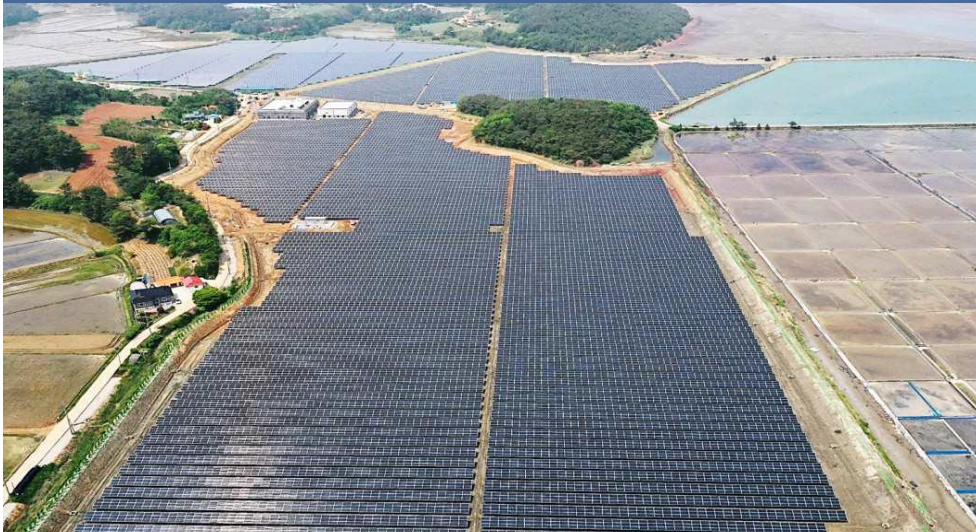
Construction of PV Power Plant in Idle Sites
