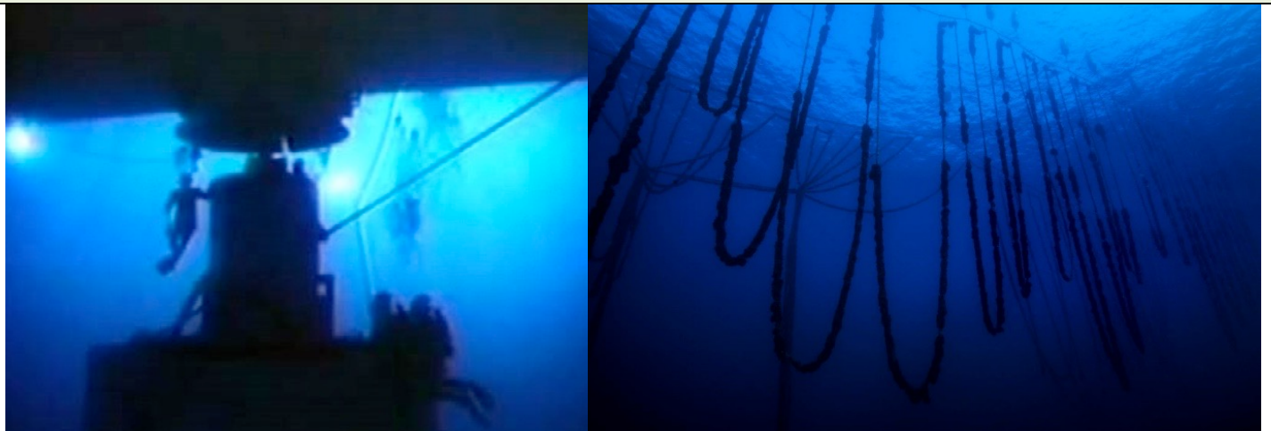
Deep-water intake pipe for no-feed multi-trophic aquaculture (design for future expansion to accommodate OTEC)
