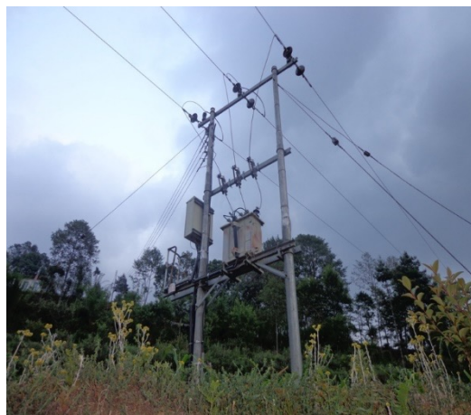
H-Pole/Transformer/11kV Line
