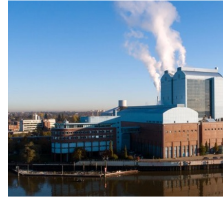
Demonstration plant Aquifer storage Tiefstack
