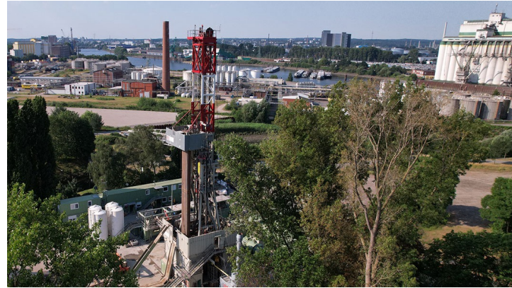
Wilhelmsburg geothermal heating centre
