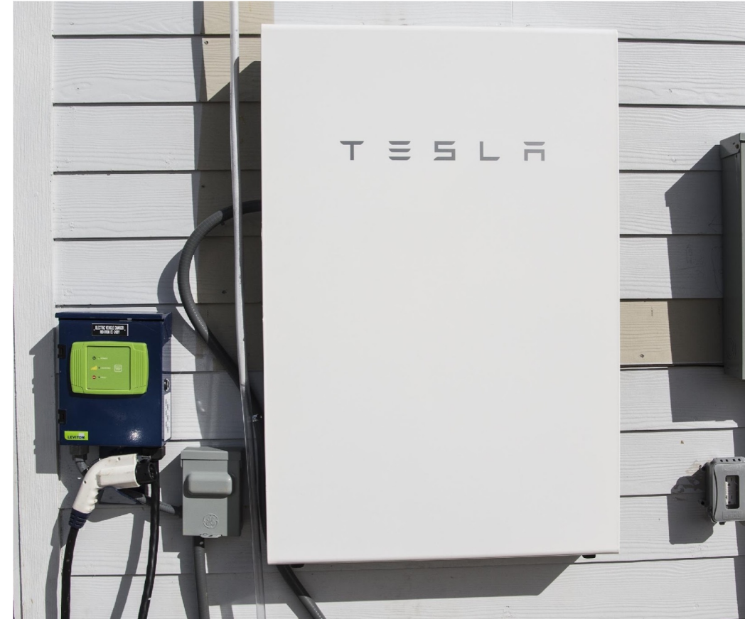
Figure. Tesla battery inverter set up: Home energy saving devices from the 2017 Solar Decathlon in Denver, CO. Dennis Schroeder/NREL. 2017.
