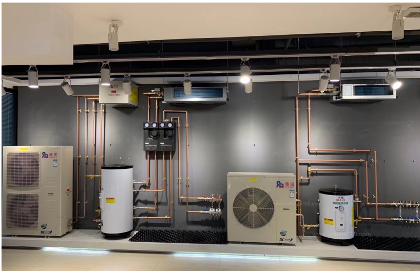
Schematic diagram of heating system of air source air-to-water heat pump
