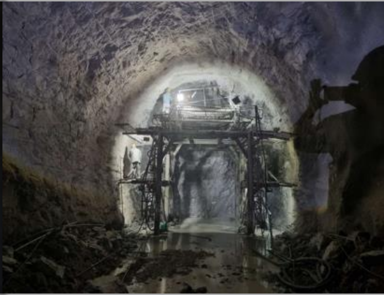
Excavation and Support Works at HRT Face 4
