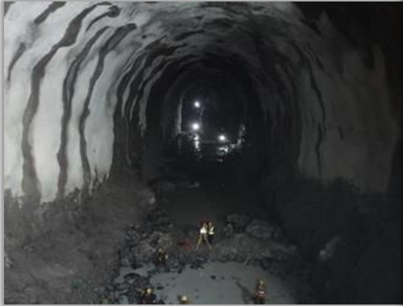
Excavation Works at Desander Main Body
