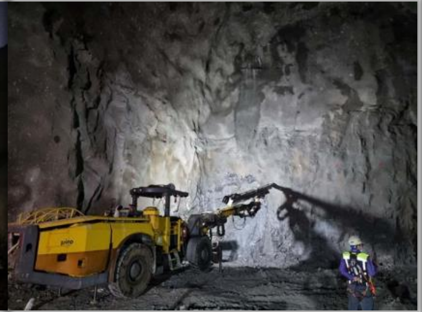
Excavation and Support works at Surge Shaft
