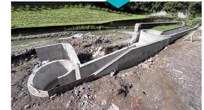
Civil work for installation of Vortex Turbines near completion
