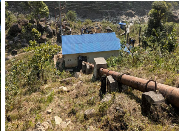
68kW Jhumsa khola MHP connected to national grid
