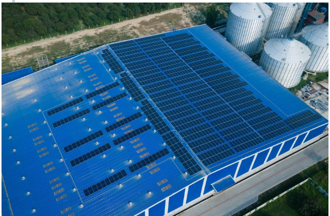
This food processing industry installed 605Kwp Solar roof-top (RESCO Model)
