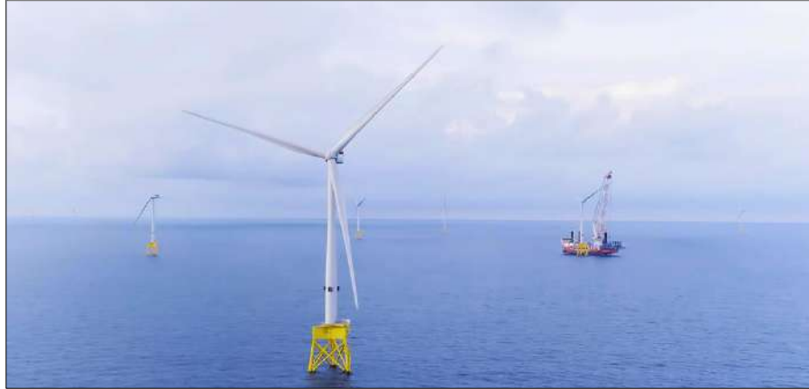
Zhong Neng wind farm 300MW completed in 2024
