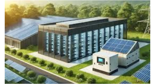
Data Centers Microgrid
