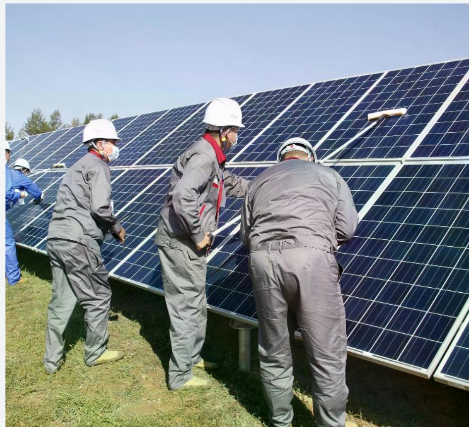
Vocational Training: PV System Installation Practical Drill
