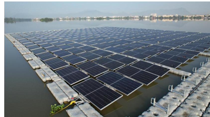
Floating solar PV at Coimbatore, India
