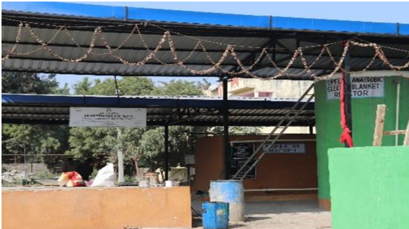
Bio-methanation Plant at Udaipur, India
