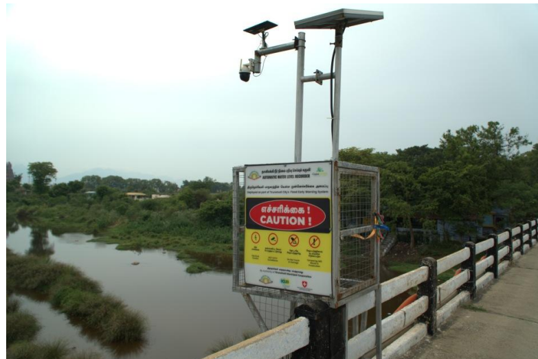
Flood Early Warning and Monitoring System at Tirunelveli, India
