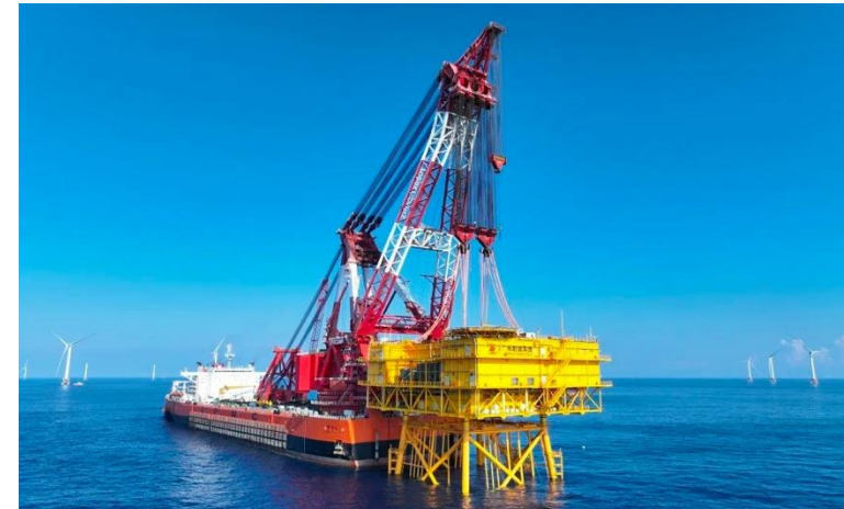
Installation of world's first 500 kV offshore AC step-up station, Yangjiang, Guangdong, 2023.
