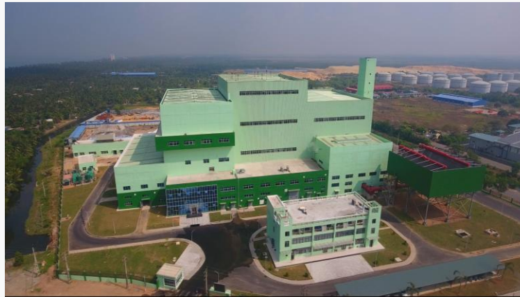
Colombo WtE Power Plant by Aitken Spence PLC
